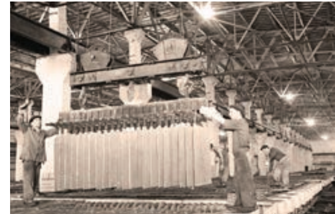
Removal of copper cathodes. Norilsk, 1956
