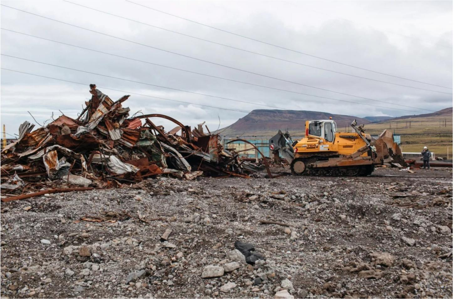
“We have removed over 5 kt of scrap metal from the cleared areas, and now we are making preparations for shipping it to the mainland for recycling. The bulk of the work will be done in the winter. In particular, we are going to cut metal constructions into several pieces so they can be shipped,” says Andrey Raduntsev, Head of Landscaping and Area Improvement at the Production Department of Nornickel’s Polar Division.
